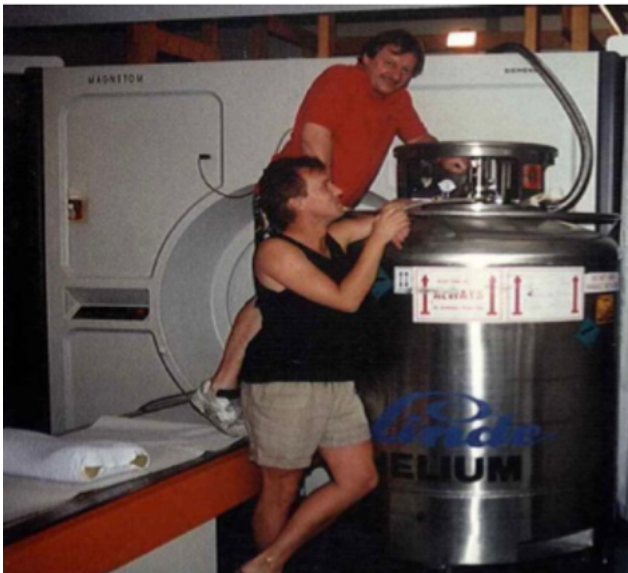
Filling of the superconducting magnet with liquid helium during the early operational phase of MRI in Würzburg. Noras was involved in the technical planning and infrastructural preparation of the facility.
